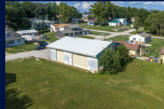
BLOCK STORAGE BUILDING
